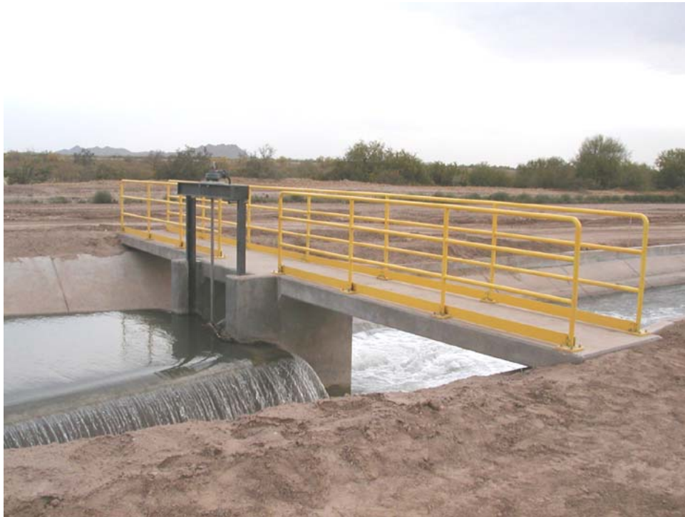
Figure 64. A check structure of this type which consists of long crested overflow weirs and a sluice gate has gained notoriety as a modern and effective check structure that can be easily automated.
