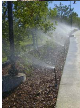
Figure 60. Typical landscape irrigation components of raw water irrigation systems. These components must be compatible with the quality of raw water.
